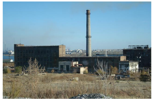
Fig. 1. General view of the former factory of acetaldehyde production.
