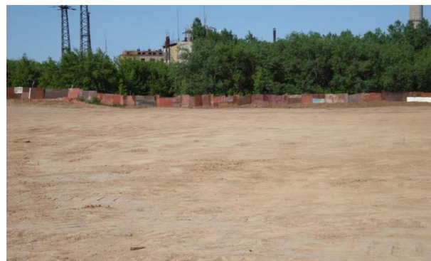
Fig. 5. The territory of the industrial site of the plant after cleaning and remediation
