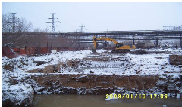
Fig. 4. Excavation of soil from the base of industrial buildings.
